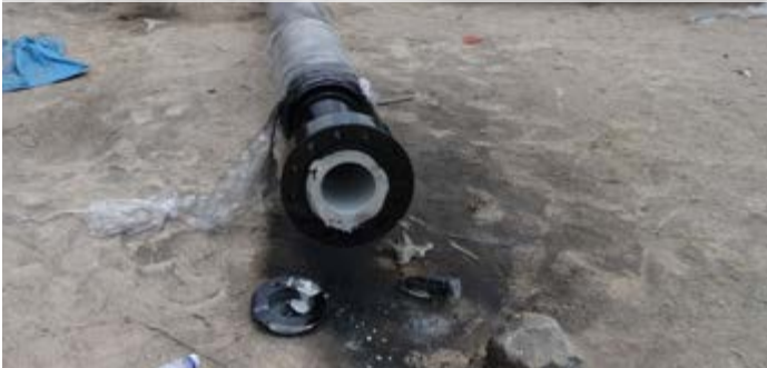
► Internal coating of pipelines for high-temperature crude oil (80 °C) – only available in English language
